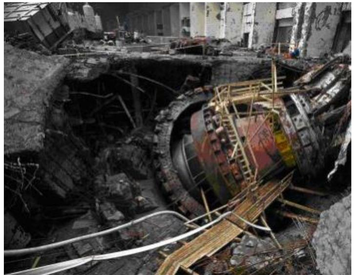
Fig. 4. View of the well of the energy unit and of the energy unit itself after the disaster
